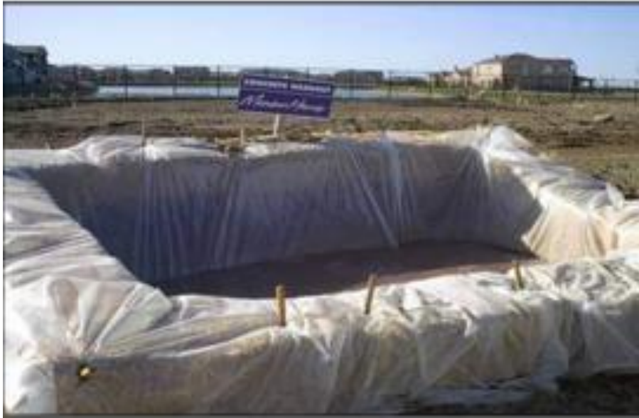
Plate 4-3 Concrete Washout Area
